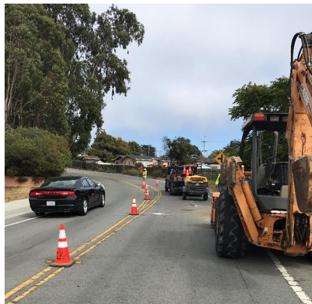
Traffic control for potholing on Coe Ave.
